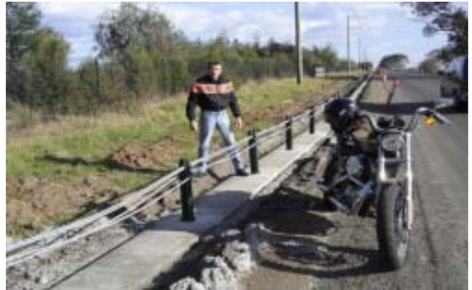
*El Presidente, Dale Maggs showing newly constructed, but as yet unfinished WRBs on one of our roads. Note the lack of clearance between the road and the WRB. Also, note the height of the WRB. How will that stop a large vehicle?*
